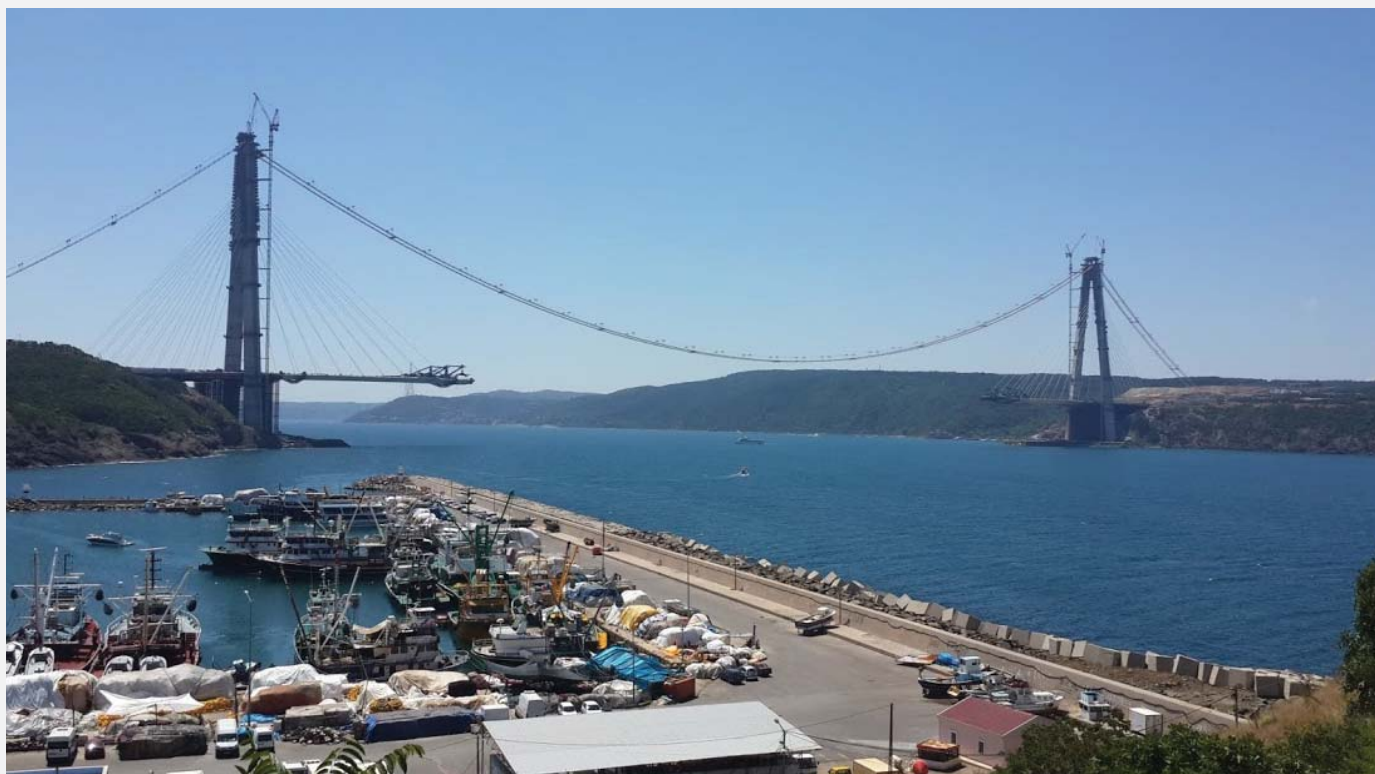
Figure 11 Progress at the Third Bosphorus Bridge in 2015 27
