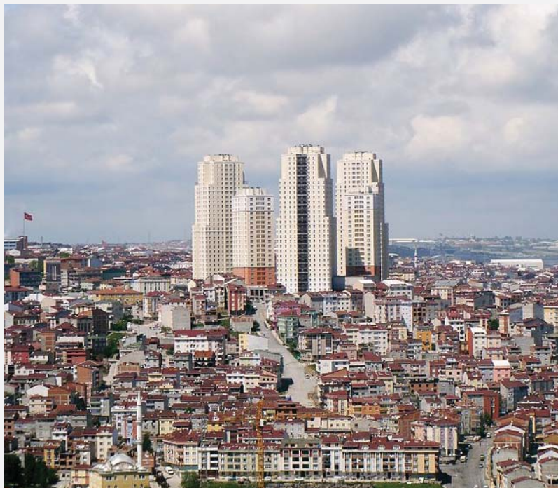
Figure 6 Gececondus and towers in Esenyurt, 25km west of Istanbul city centre 5
