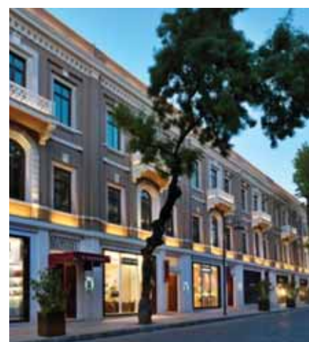
Renovated building façade at Akaretler; courtesy of the Bilgili Group © 2009
