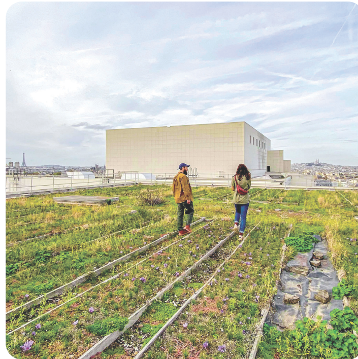
Opéra Bastille rooftop in Paris Topager, 2017
