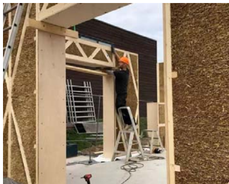
Straw school building, Felballe Friskole
